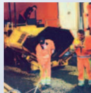
■ Road construction workers build a sample of Icelandic road at a Swedish research institute, where extensive tests were carried out on Icelandic road materials.
